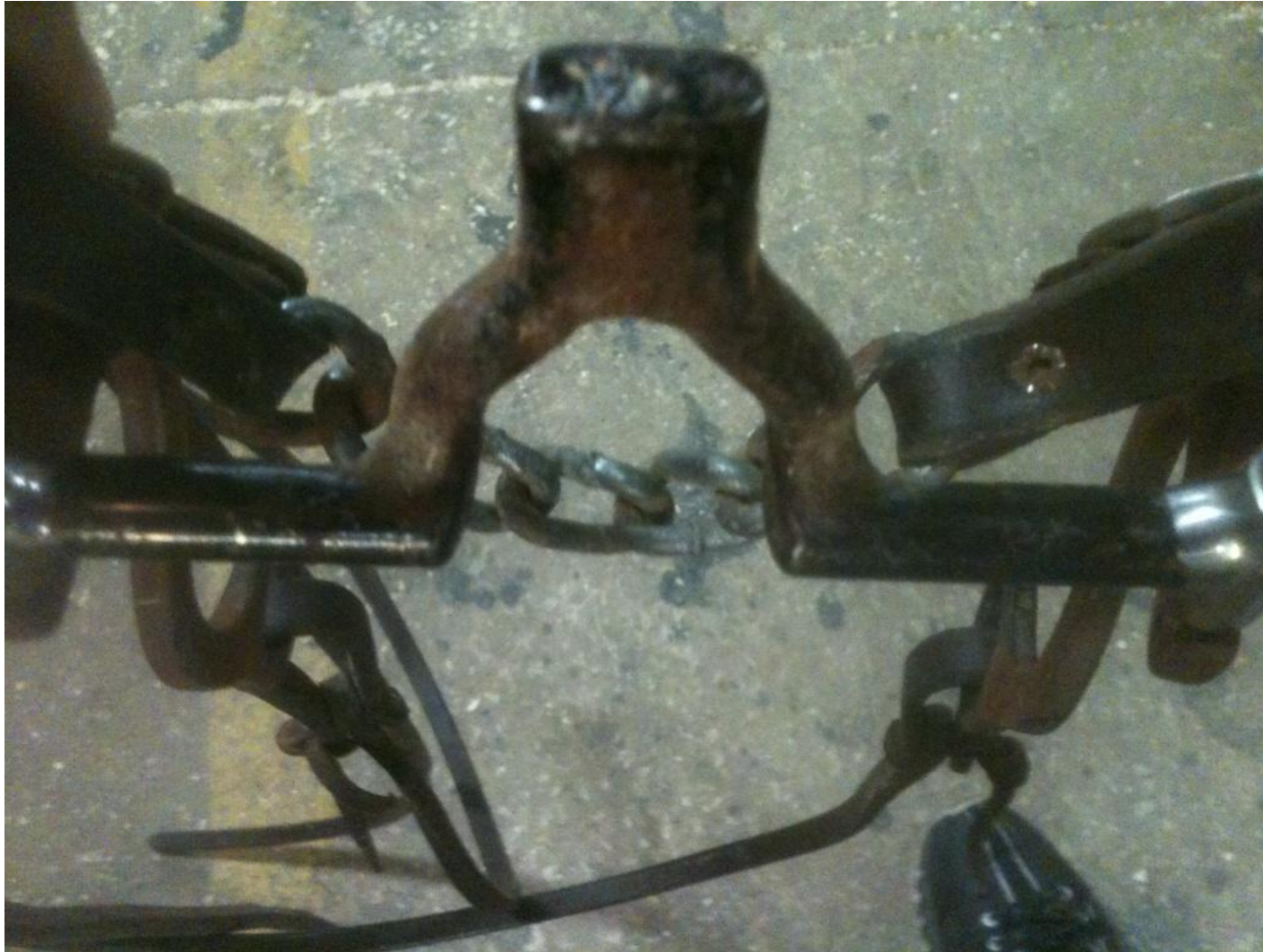
Illegal – Off Set Port
